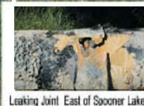
Leaking Joint East of Spooner Lake
